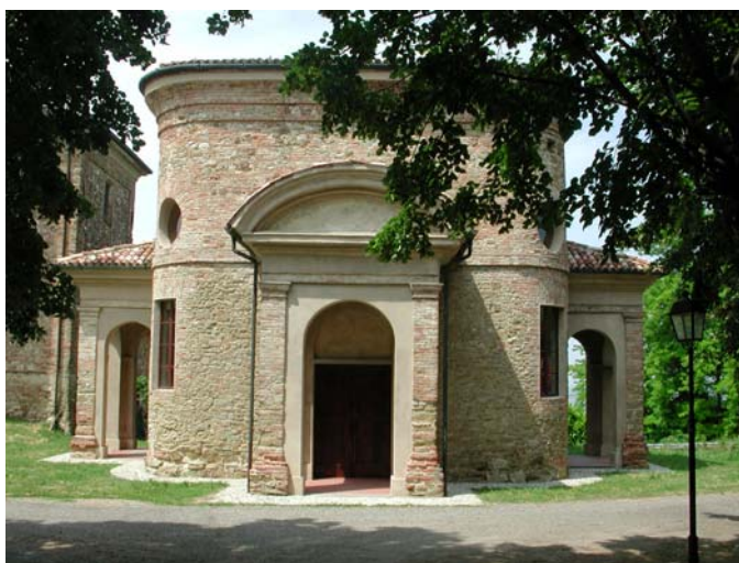
Foto: Architecture Workshop Miconi & Partners
